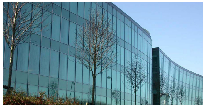
The Quadrant Cobalt Business Park; North Tyneside Council's new offices and data centre
